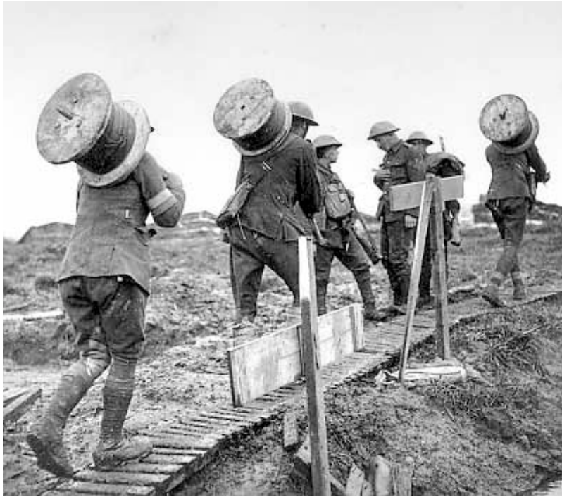
Figure 11. Official Photograph Taken on the British Western Front in France. The Battle of the Ridges. Telegraph wire going up for No Man's Land. Signallers on the way to establish communications. [Original Title] (John Warwick Brooke. First World War 'Official Photographs,' no. D. 2114. National Library of Scotland).
