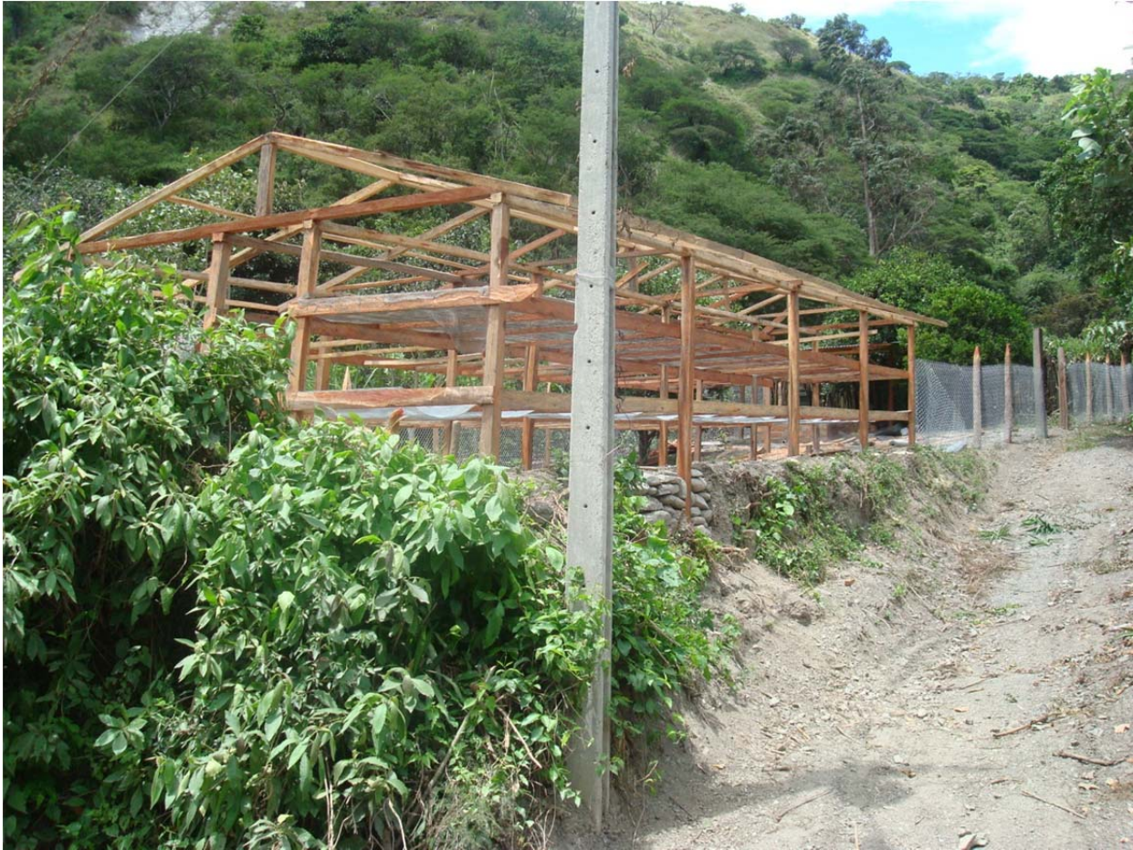
Figure 15. A marquesina in construction
