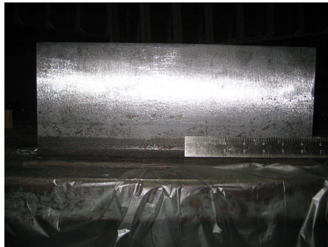
Figure 3.4 Representative photo of steel surface prepared for FRP application.
