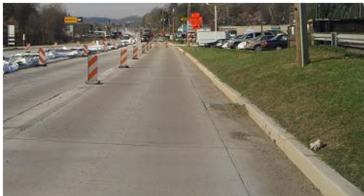
Figure 3.5 Test section in the westbound lanes.
