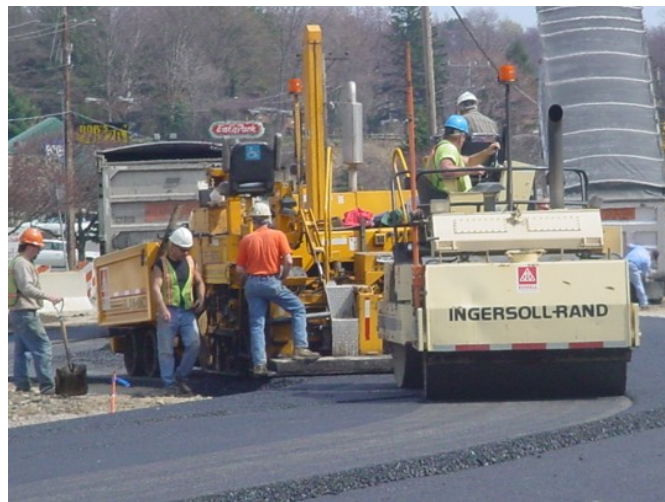
Figure 3.14 Placement of the ATPB.
