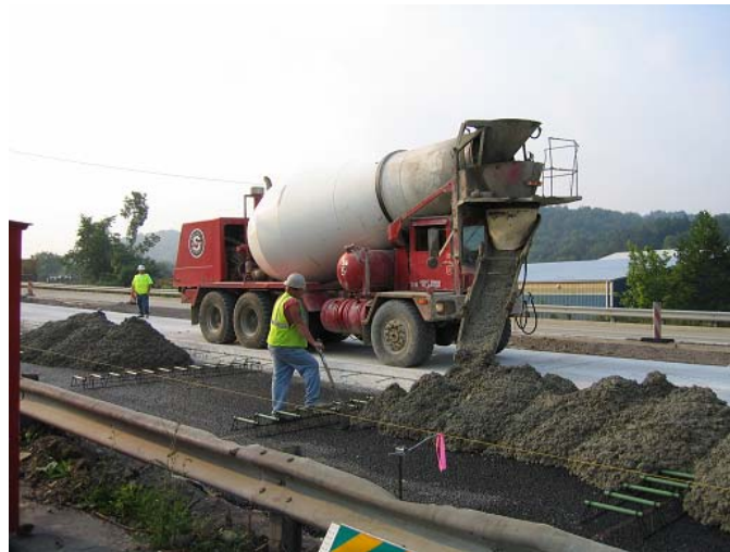
Figure 3.20 Concrete truck delivering fresh concrete to site.
