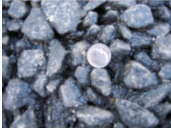
Figure 3.13 Close up of the ATPB prior to placement of the concrete.
