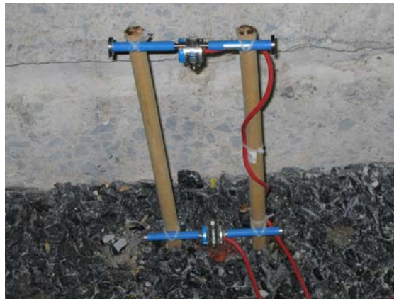
Figure 3.28 Static strain gage installation.
