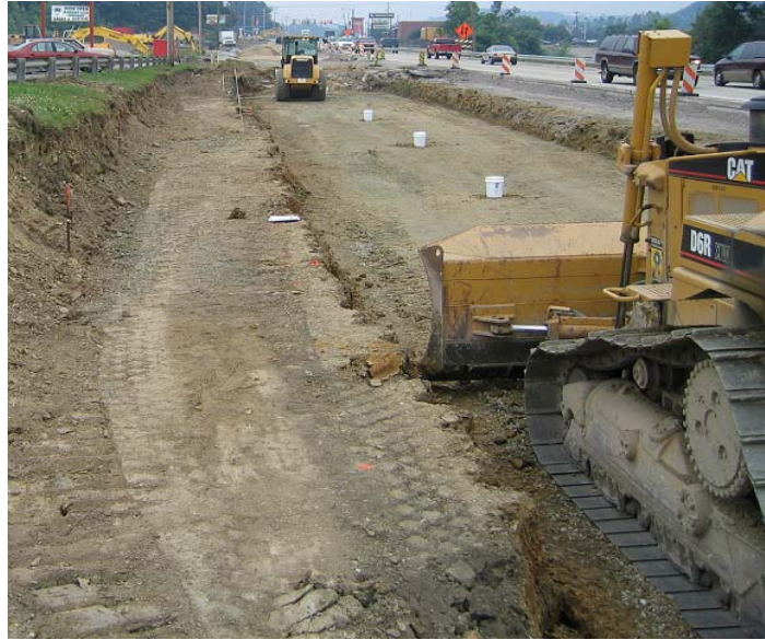
Figure 3.9 Excavation of existing subgrade.
