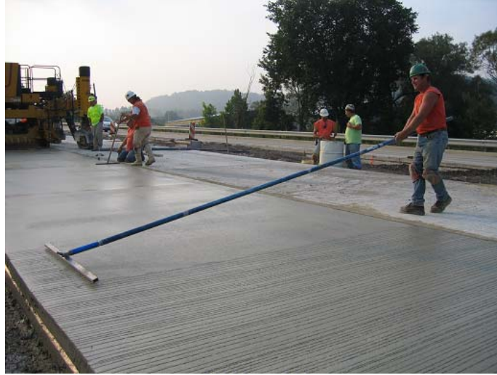
Figure 3.22 Application of transverse tining.
