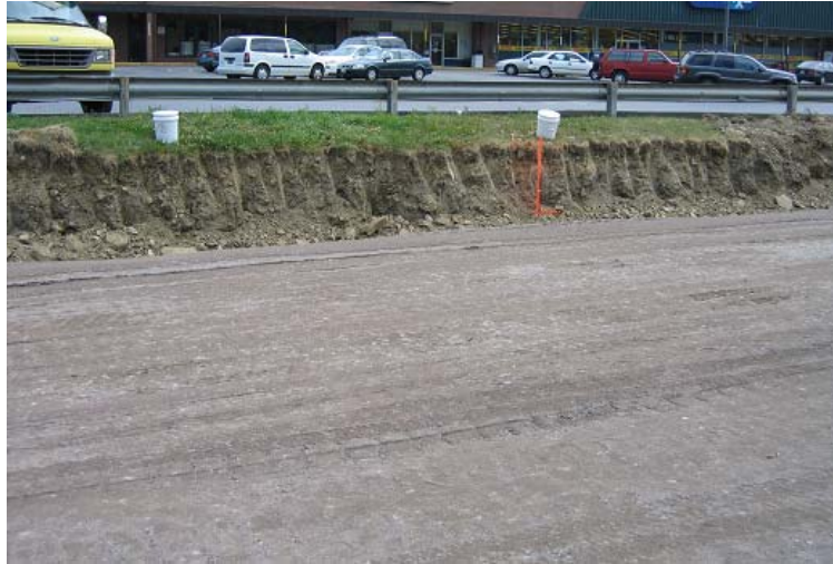
Figure 3.12 Slag subbase placed on top of the fill material.
