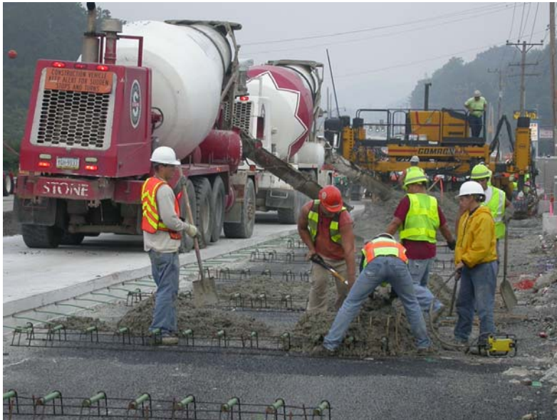
Figure 3.21 Concrete was hand placement around the sensors.
