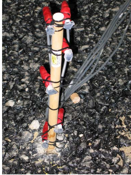
Figure 3.27 Installation of relative humidity sensors.
