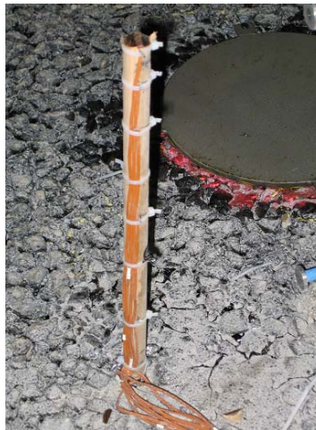
Figure 3.23 Temperature sensor installation.
