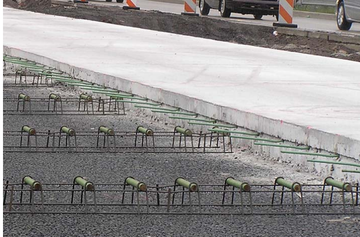
Figure 3.7 Dowel and tie bar configuration on SR-22.
