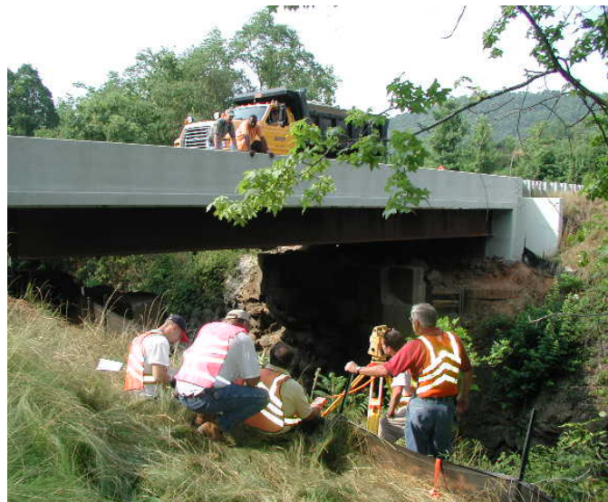
(c) photograph of South Carolina SC655 Bridge
