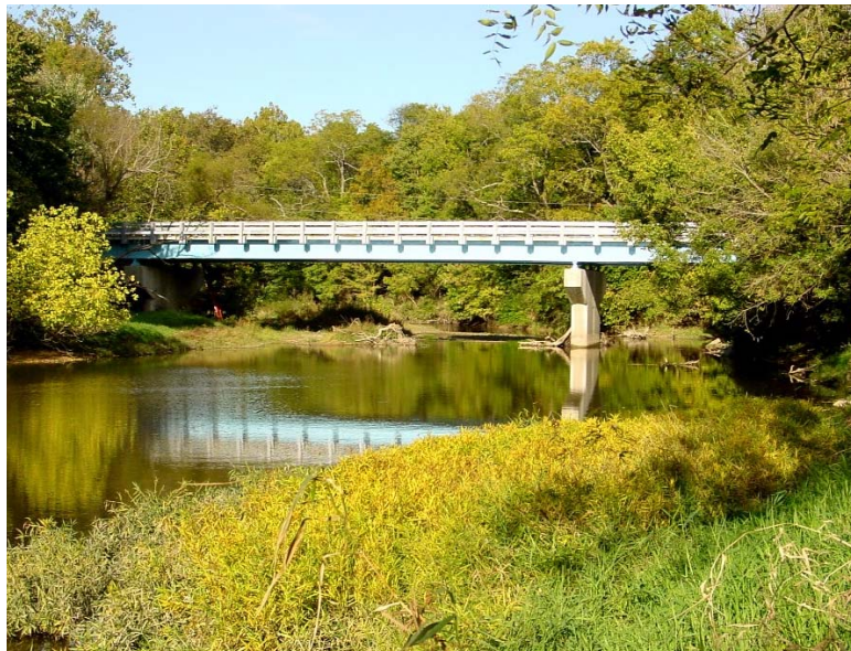
(c) photograph of Fairground Road Bridge
