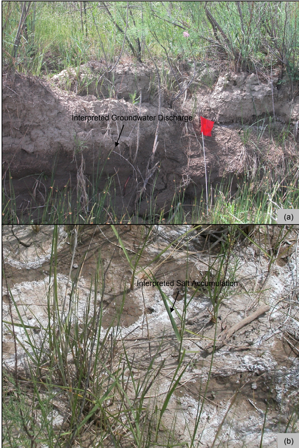
Figure 5.9. Field photographs of apparent groundwater discharge along the Powder River bank downgradient of the NC7 produced water disposal impoundment. (a) View of the bank approximately 3 m from stream with interpreted groundwater discharge. (b) White crust interpreted to be accumulated salts adjacent to (a). Photograph by James Sams.
