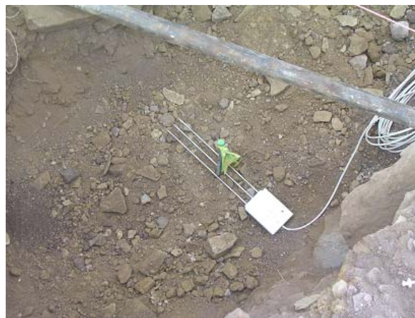
Figure 3.11. Installation of CS605L TDR probe in the subgrade (Wells et al. 2005).
