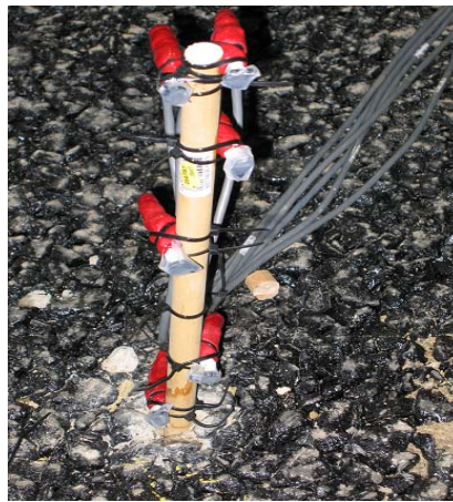
Figure 3.8. Relative humidity sensors located throughout the PCC slab (Well et al. 2005).
