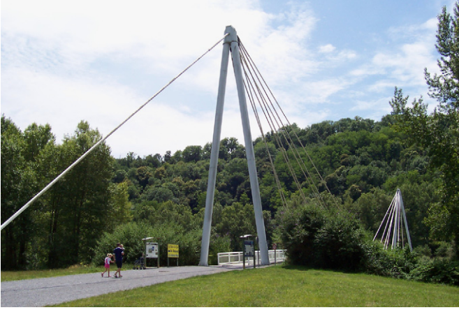
Fig. 1. The Laroin footbridge (France, Pyrénées Atlantiques).
