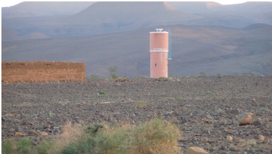
(B2) SAEP Water Tower of 'Àfra, Ouled Ahmed ben Ali and Zaouite ben Talib
