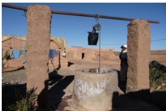
Figure 4.1: Typical Draw Well, 'Àfra
