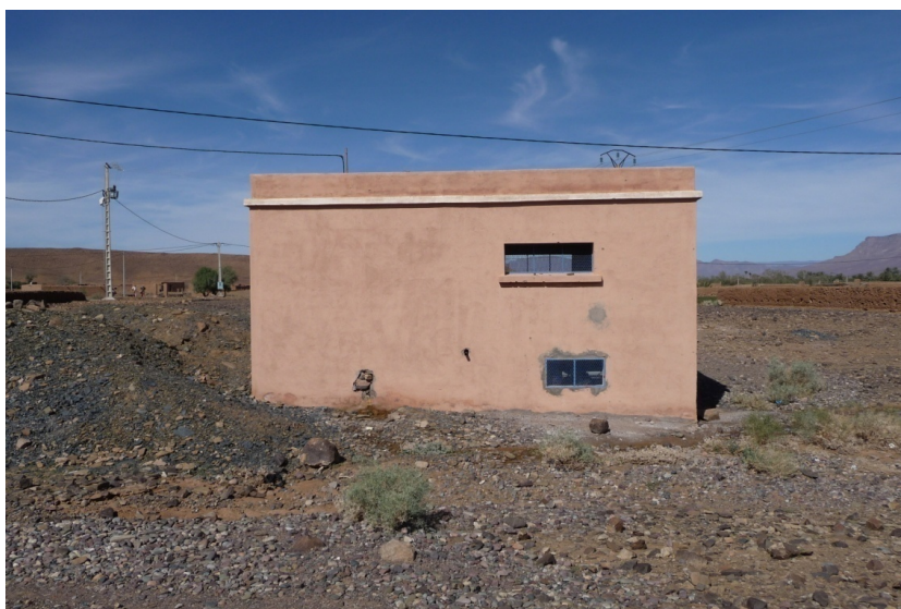
(B6) SAEP Electric Pump and Well in Cement Building in Qsbat al-Ghamàd
