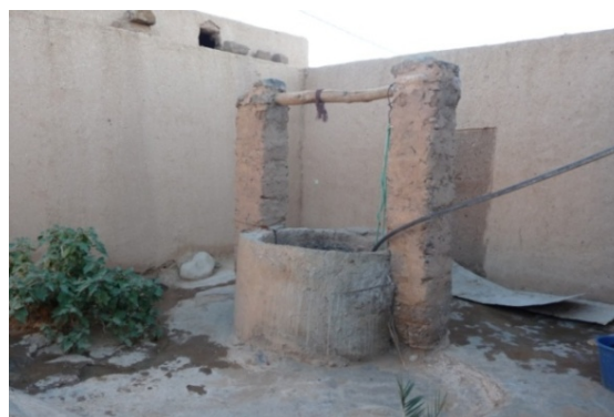
Figure 4.2: Well with Electric Pump, 'Àfra
