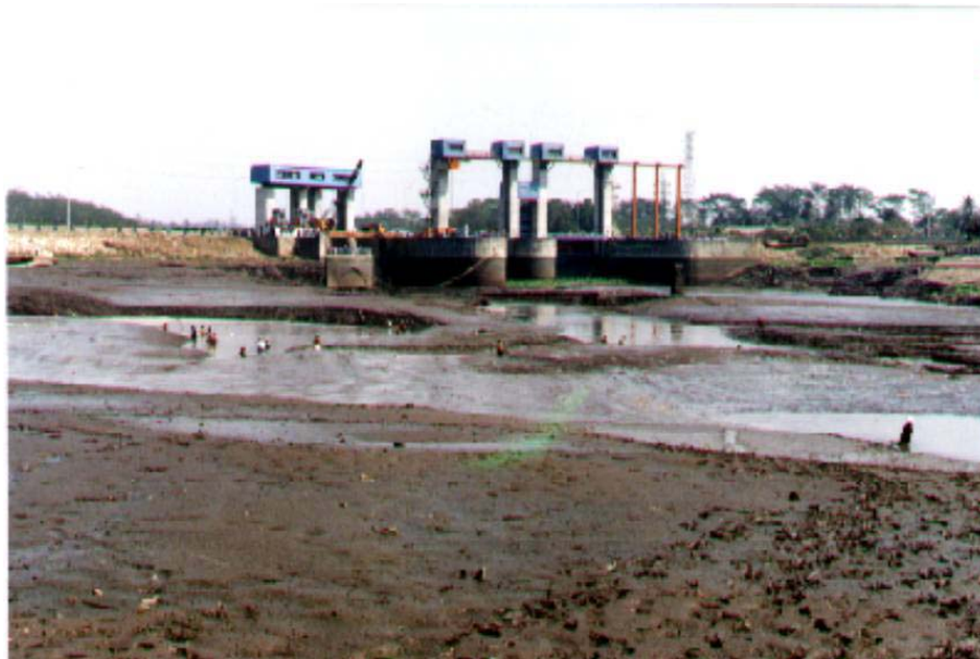
Figure 2: Sedimentation of the Sengguruh reservoir in East Java, 2000
