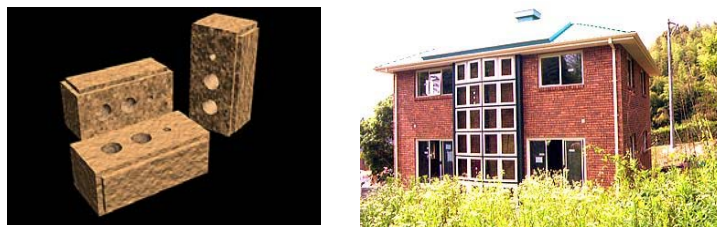
Figure 7. Double storey DBHS Experimental House and 3D-view of clay bricks used in the project.
