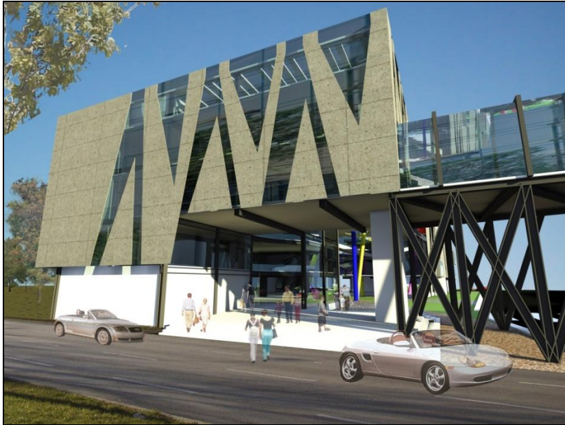
Figure 15: The green design implementation on the façade of the library using perforated panels and AAC panels [6]
