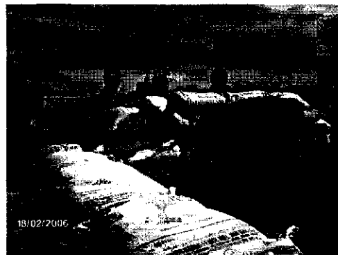
8) Arrange the sandbag close to the door frame
