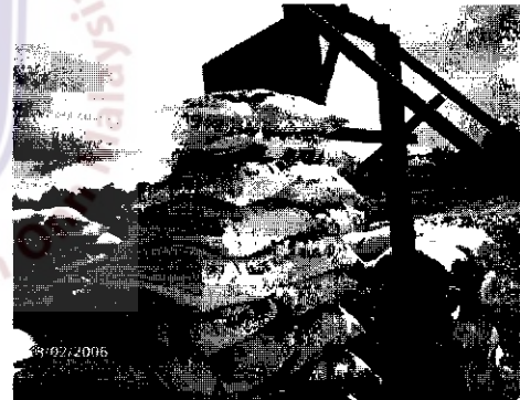
8) Arrange the sandbag close to the door frame
