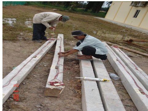
Fig. 2: Installing the strain gauge prior to driving
