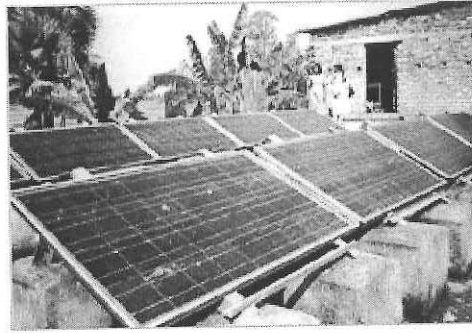
Figure 2.6 Photovoltaic (PV) modules are composed of multiple PV cells.[10]
