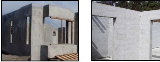
Figure 5: Foamed concrete as blocks and wall panels.
