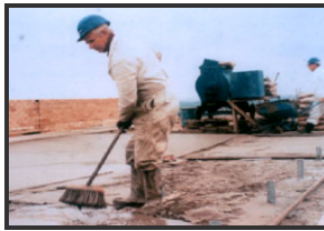
Figure 6: Application of foamed concrete as roof insulation material
