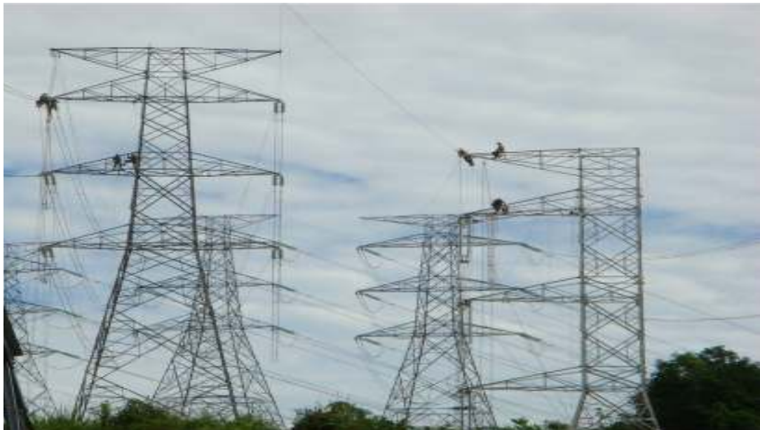
Figure 1.1 : Maintenance at Transmission Lines
