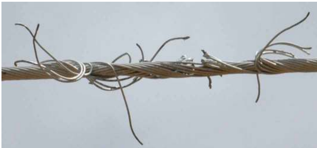
Figure 2.6 : Conductor damage due to vandalism resulting in broken strands and exposure of core.
