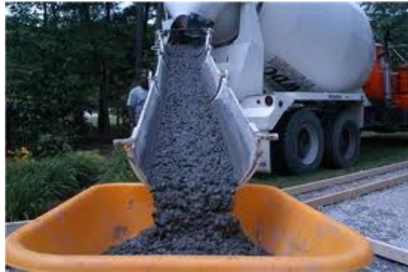
Figure 2.2: Ready-mixed concrete from truck ( www.concretenetwork.com )
