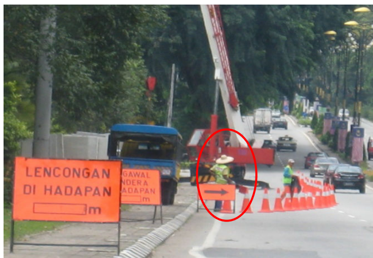
Figure 1. The flagman is placed in the road construction work zone
