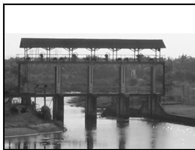
Figure 1: Sluice Gate Location at Sungai Sembrong in Parit Raja
