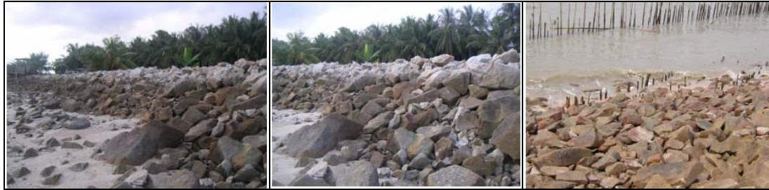
Figure 6: The condition of revetment at the area.
