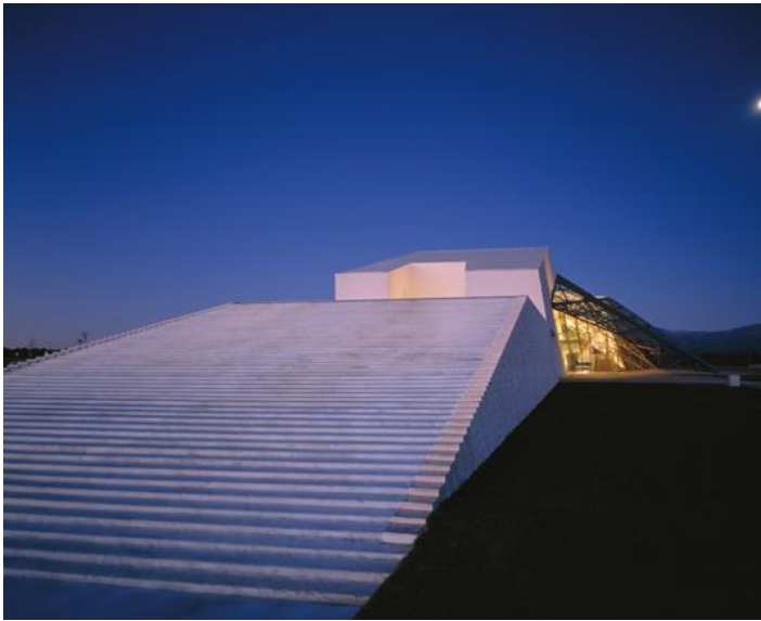
Fig.21, Spencer Theater, the sloped roof (Alto, 1998)
