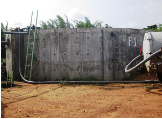
Figure 3.6. The effluent is taken out through the overflow shaft.
