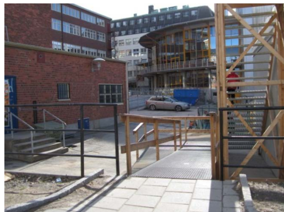
Fig. 30 – Stairs and ramps close to Fryshuset.
