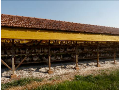
Figure 8. No walls were present at the animal facilities. The construction was made of wood. (Photo: Caroline Olofsson)
