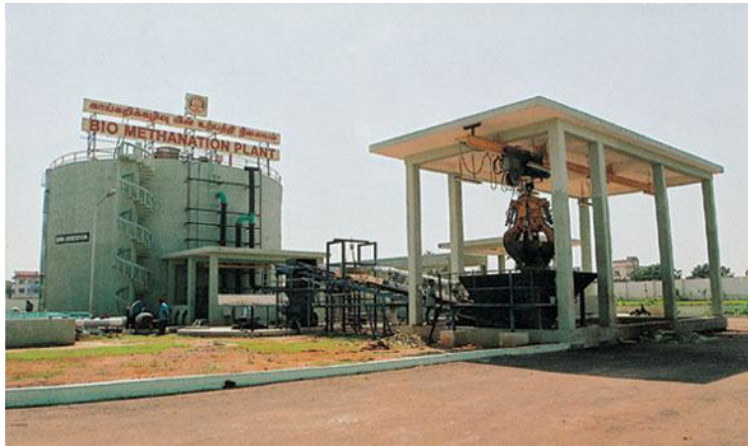
Figure 3 The biomethanation plant in Koyembedu wholesale market complex, Chennai. [57]
