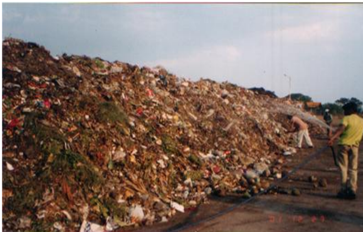
Figure 21 Bioculture is sprayed on the windrows. [37]
