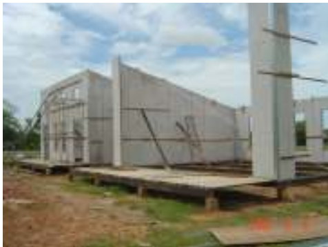
Figure 8(c). The propped wall and laid floor panels
