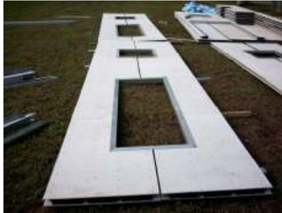
Figure 5: Double skin wall panel with window openings
