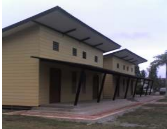
Figure 9: Completed classroom modules
