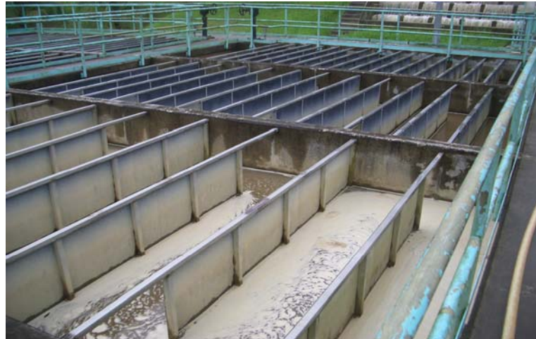
Plate 2.2: Three stages of baffles type flocculation tank (With permission from the Segama WTP)
