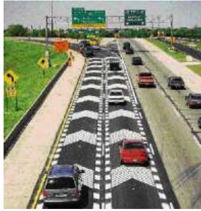
Figura 2-19 – Convergenza Chevron Milwaukee County, Wisconsin (Rothenberg et al., 2004)
