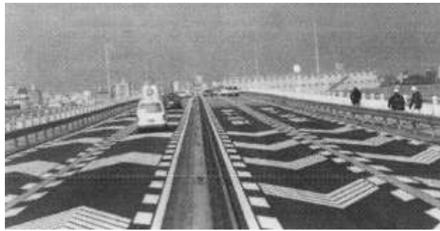
Figura 2-17 – Convergenza Chevron ponte Yodogawa, Japan (Meyer, 1999)
