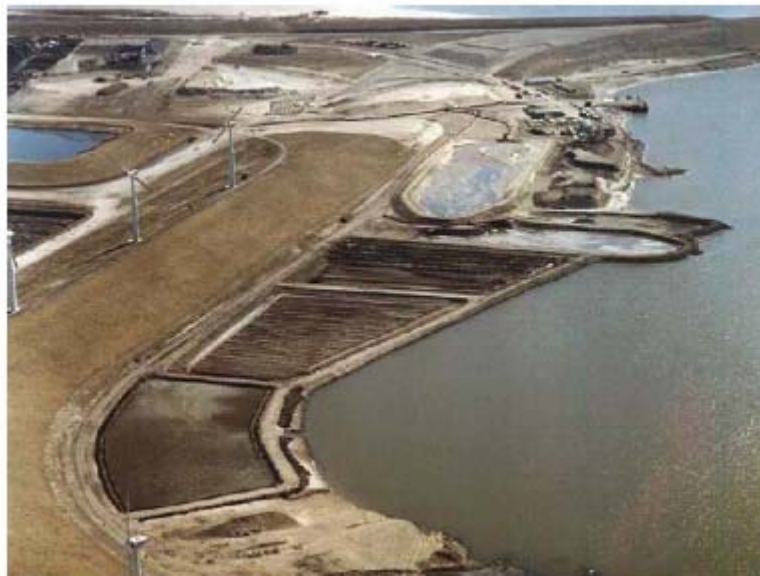
Figure 3.1. Slufter with dewatering fields and sedimentation basins
