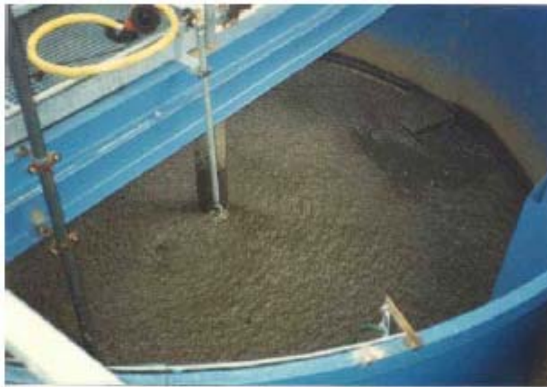
Figure 3.4. Bioreactor used for the degradation of oil and PAH in dredged material
