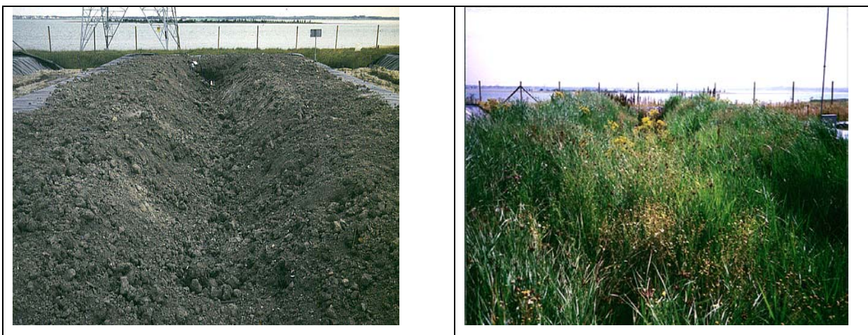
Figure 3.3. The Petroleum Harbour landfarms on Kreekraksluizen. Left the cultivated landfarm in 1995. Right the vegetated landfarm in 1997 (from Harmsen 2004)
