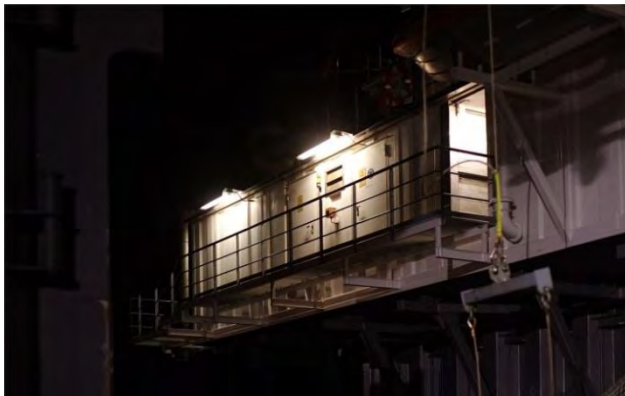
Figure 7: Deployment of light guidance shields on standby electricity generator (Photograph: Studio B8 on behalf of RWE Dea AG).
