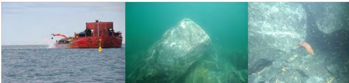
Figure 2: Left: Boulder dumping in 2008. Middle and right: pictures of the new reef at Læsø Trindel in 2008.
