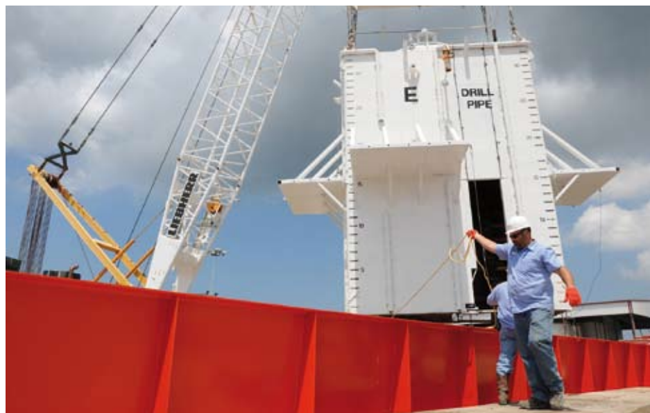
Abb. 1 | PORT FOURCHON, La. - Crewmen aboard the motor vessel Joe Griffin guide a cofferdam onto the deck as the ship prepares to depart Wild Well Control May 5, 2010. The chamber was designed to contain the oil discharge, that was a result of the „Deepwater Horizon“ incident, before it reaches the surface. © U.S. Coast Guard photo by Petty Officer 3rd Class Patrick Kelley.
