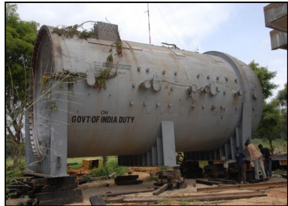
Figure 11. Erection of the shell at the site
