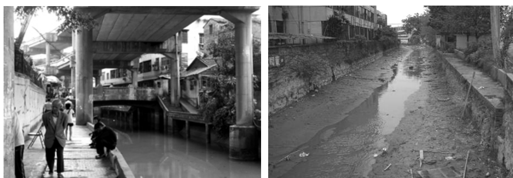
the deteriorated water system in Guangzhou and Foshan
