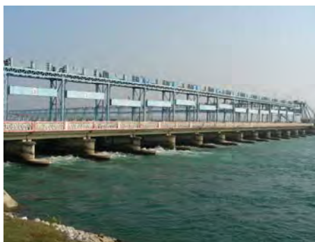
Girijapuri Barrage, KAT
