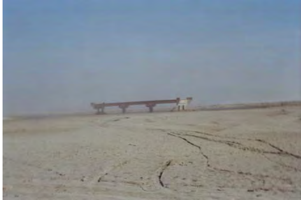
Old Sharda Bridge. Due to change in course of river and excessive silt, bridge is now abandoned.
