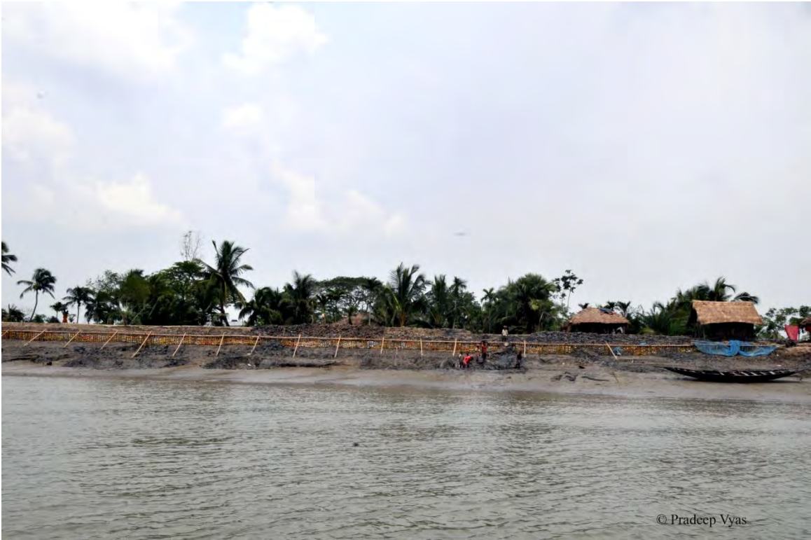
Plate 9: Earthen embankments to protect villages from tidal water
