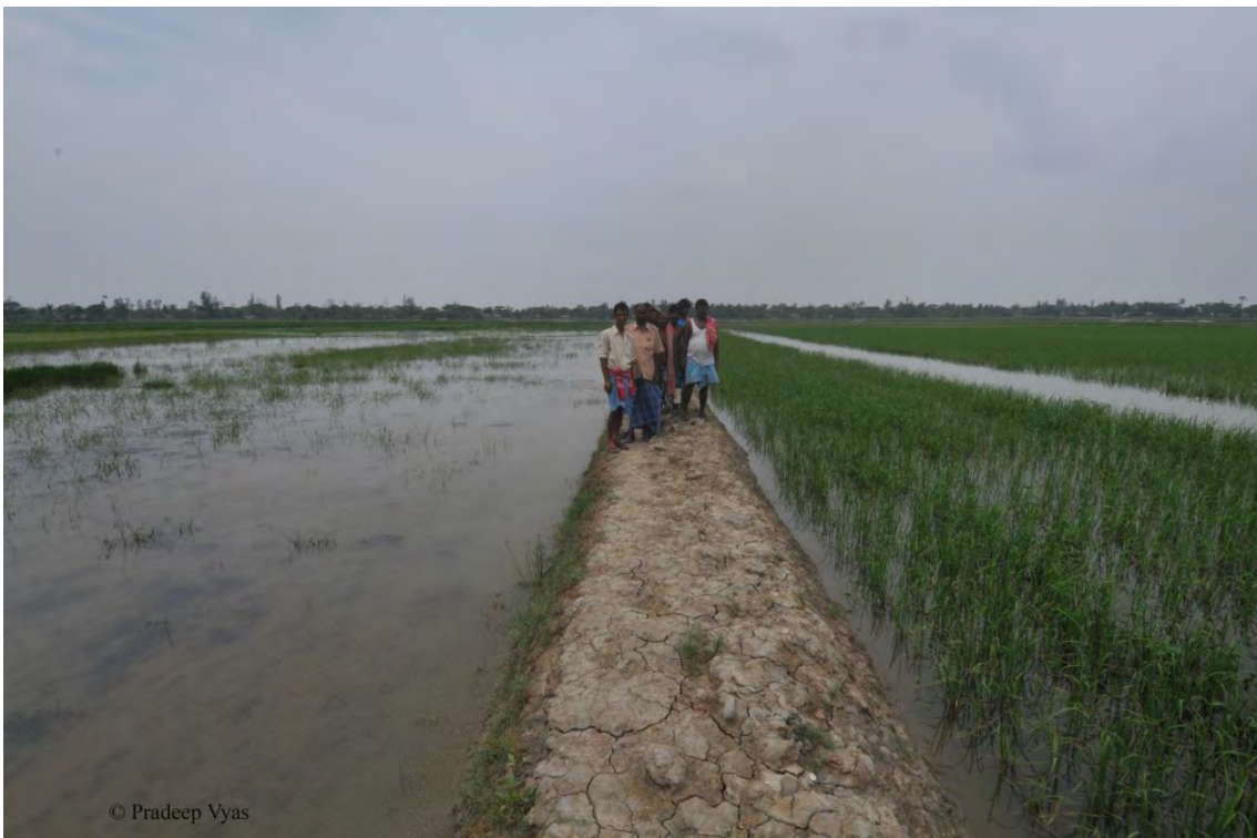
Plate 10: Flooding of saline water due to breach of embankment
