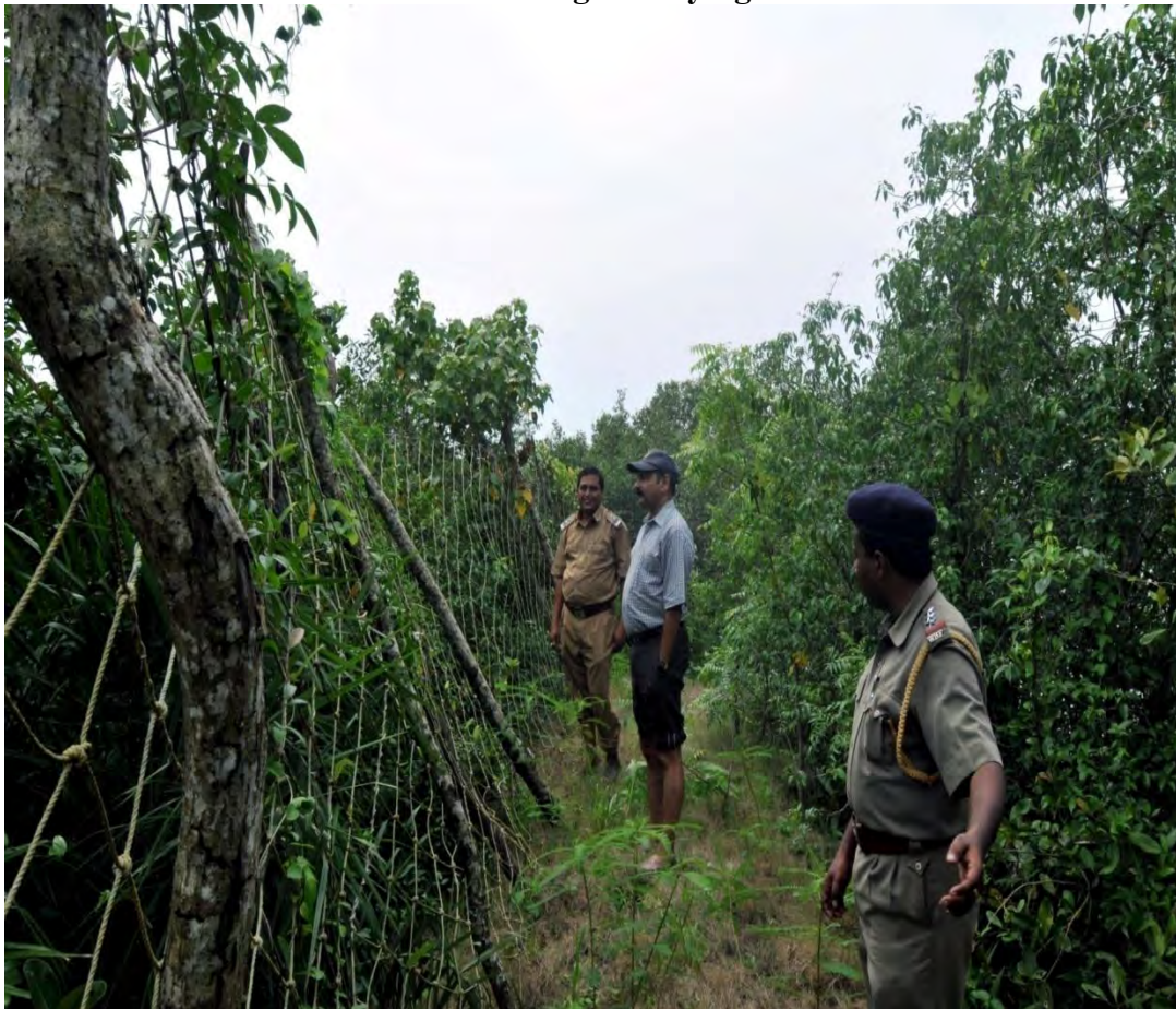
Plate 28 a: A poorly maintained “Nylon-net fence”
