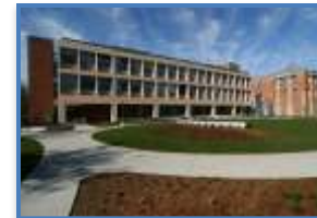
CAMCOR is located in the Lorry Lokey Science Complex, University of Oregon
