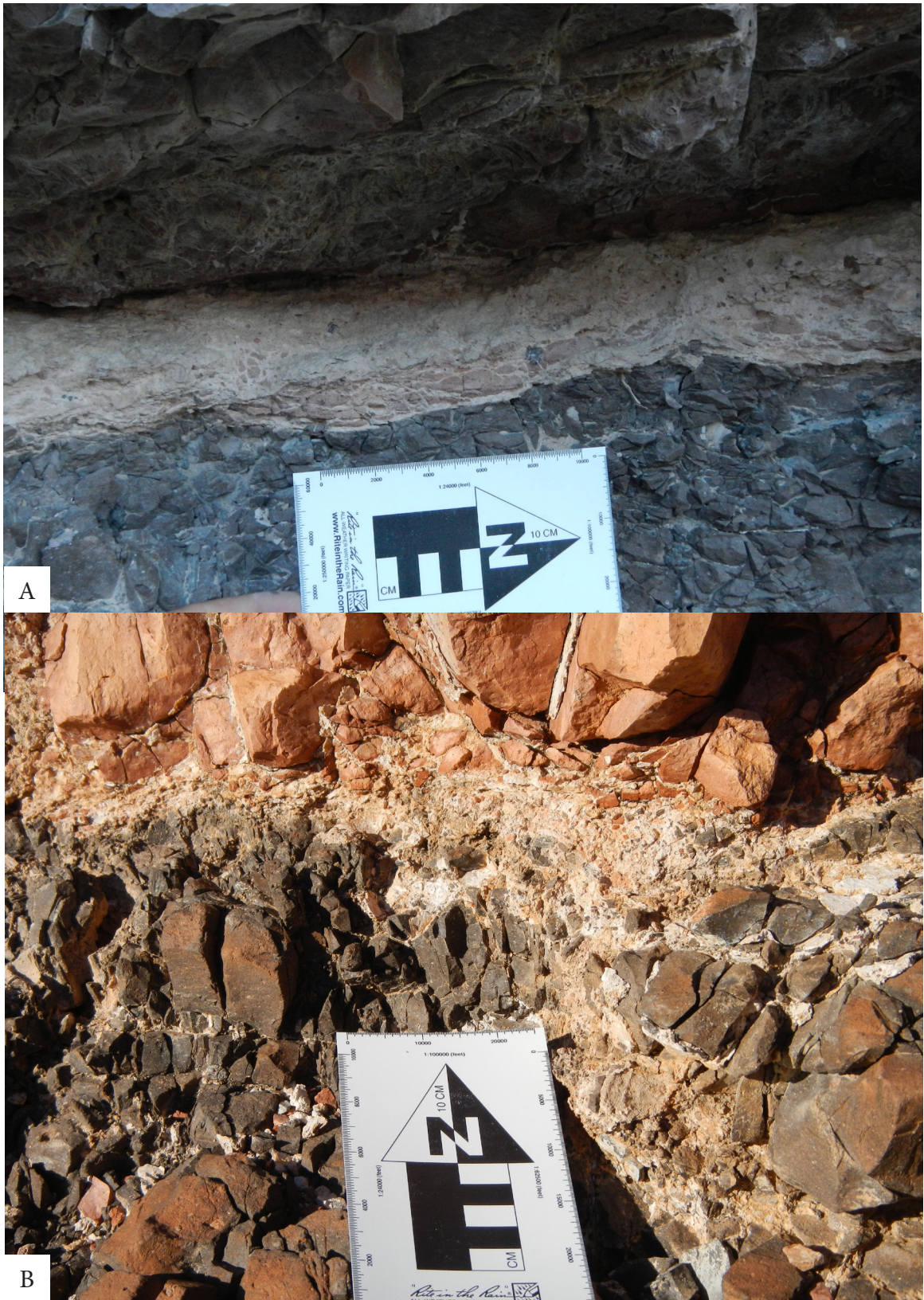
Figure 4. Close-up of fault contacts
