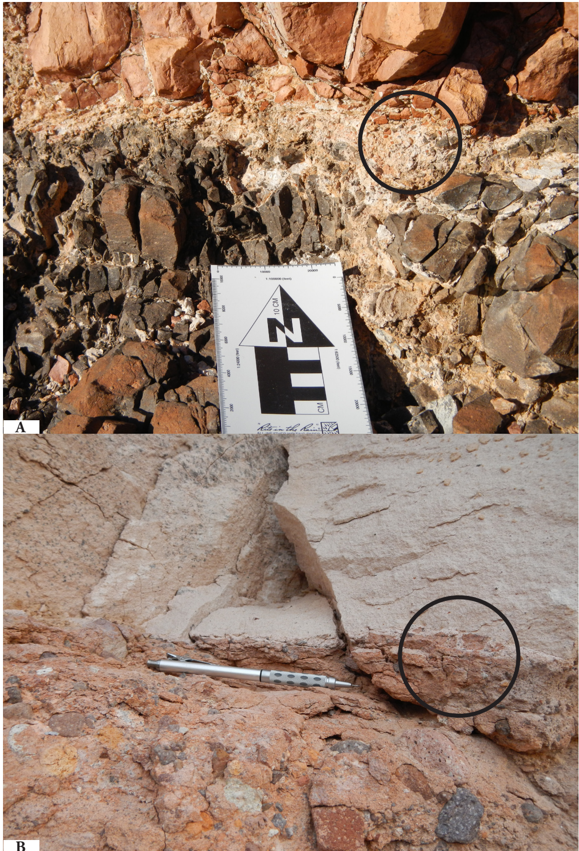
A B Figure 19. Fault vs depositional contact
