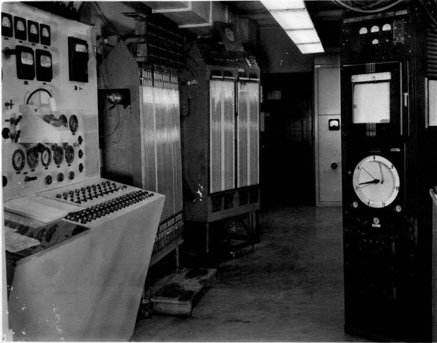
SECTION OF GALCIT HYPERSONIC WIND TUNNEL CONTROL ROOM
