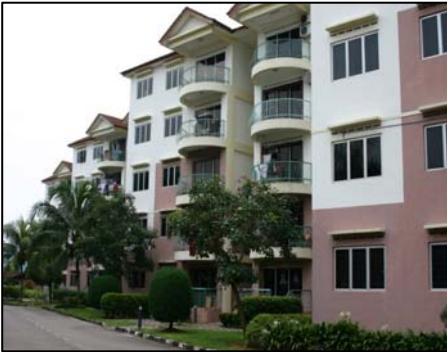
Figure 8: Sample building for the experiment purposes
