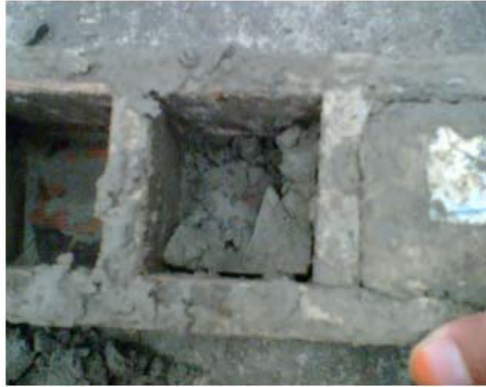
Figure 4.3: Crumbles of 50% EM-AS Cement Cube at day 3
