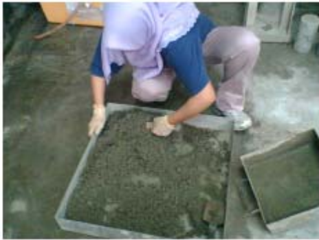
Figure 3.7: Preparing the Mortar Mix
