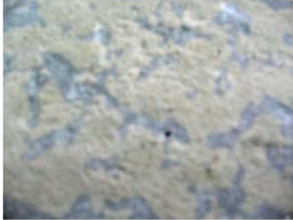
Figure 4.29: The Closer Look at the Surface of 100% EM-AS Concrete Cube
