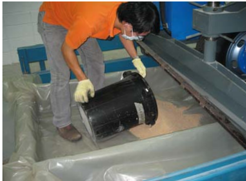
Figure 4: Screeding bedding sand
