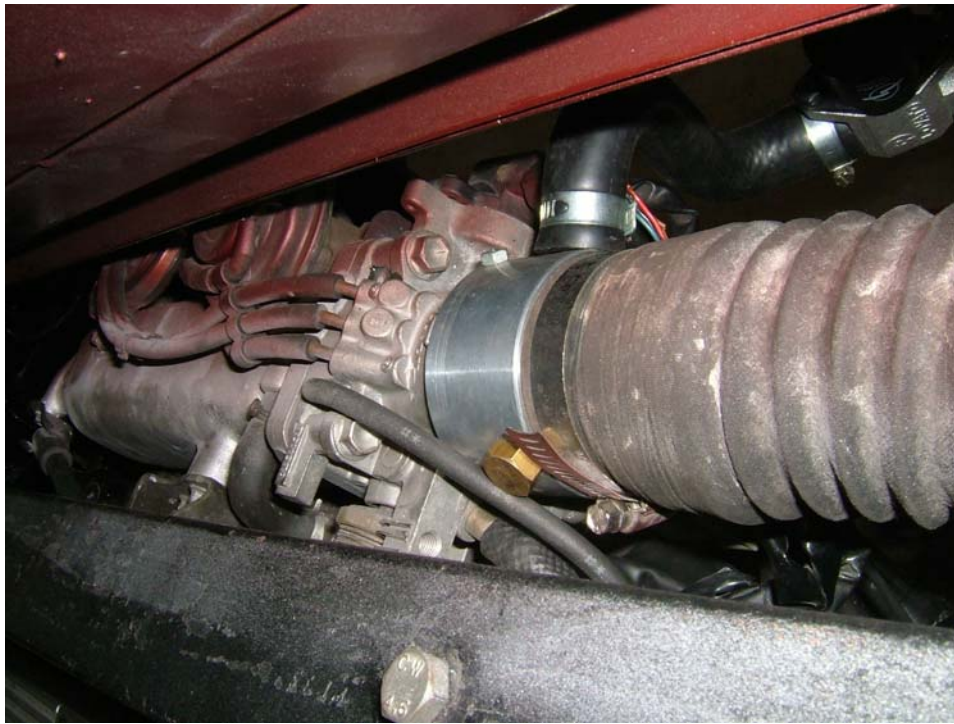
Figure 6.17: Installation of the mixer to the air intake manifold and the CNG supply line
