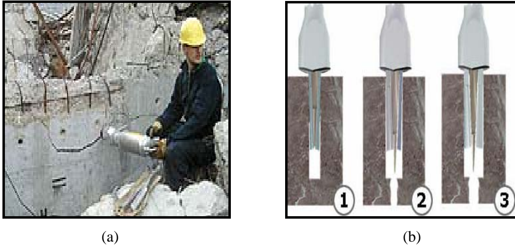
Figure 2.8: (a) A hydraulic splitter, (b) Mechanism of operation (www.darda.de, 2005).
