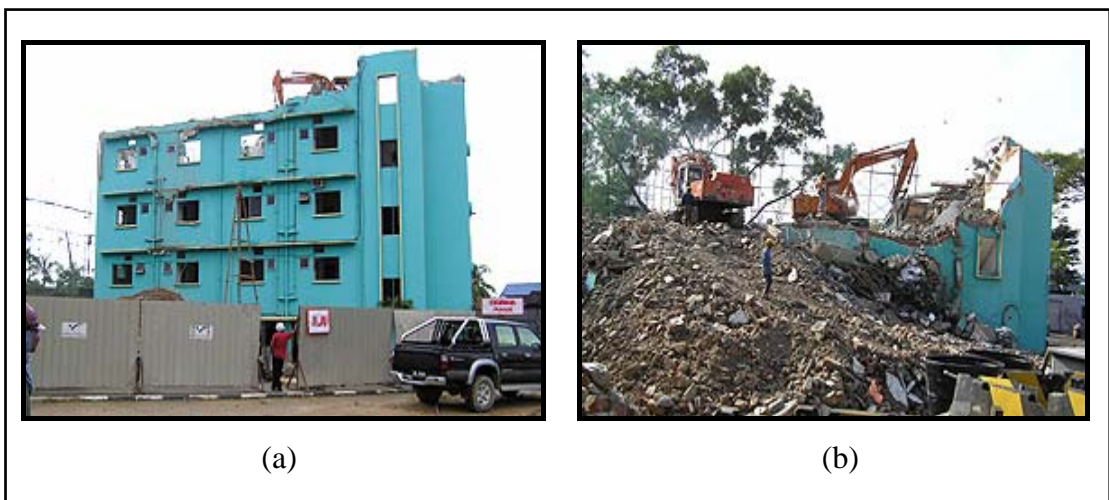
Figure 4.3(a-b): Demolition of Malaya Hotel in progress.
