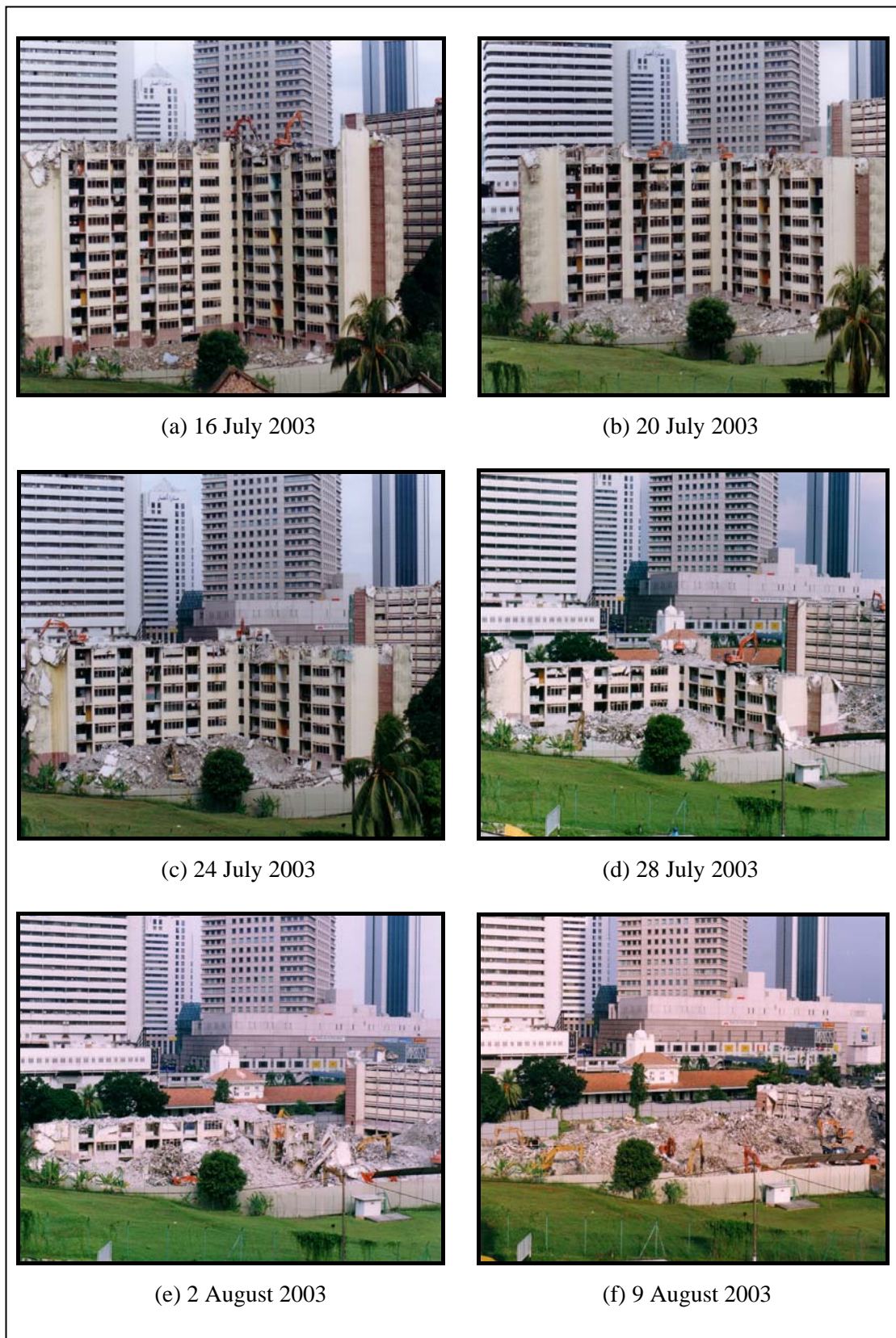
Figure 4.10 (a-f): Demolition operations at Block B.
