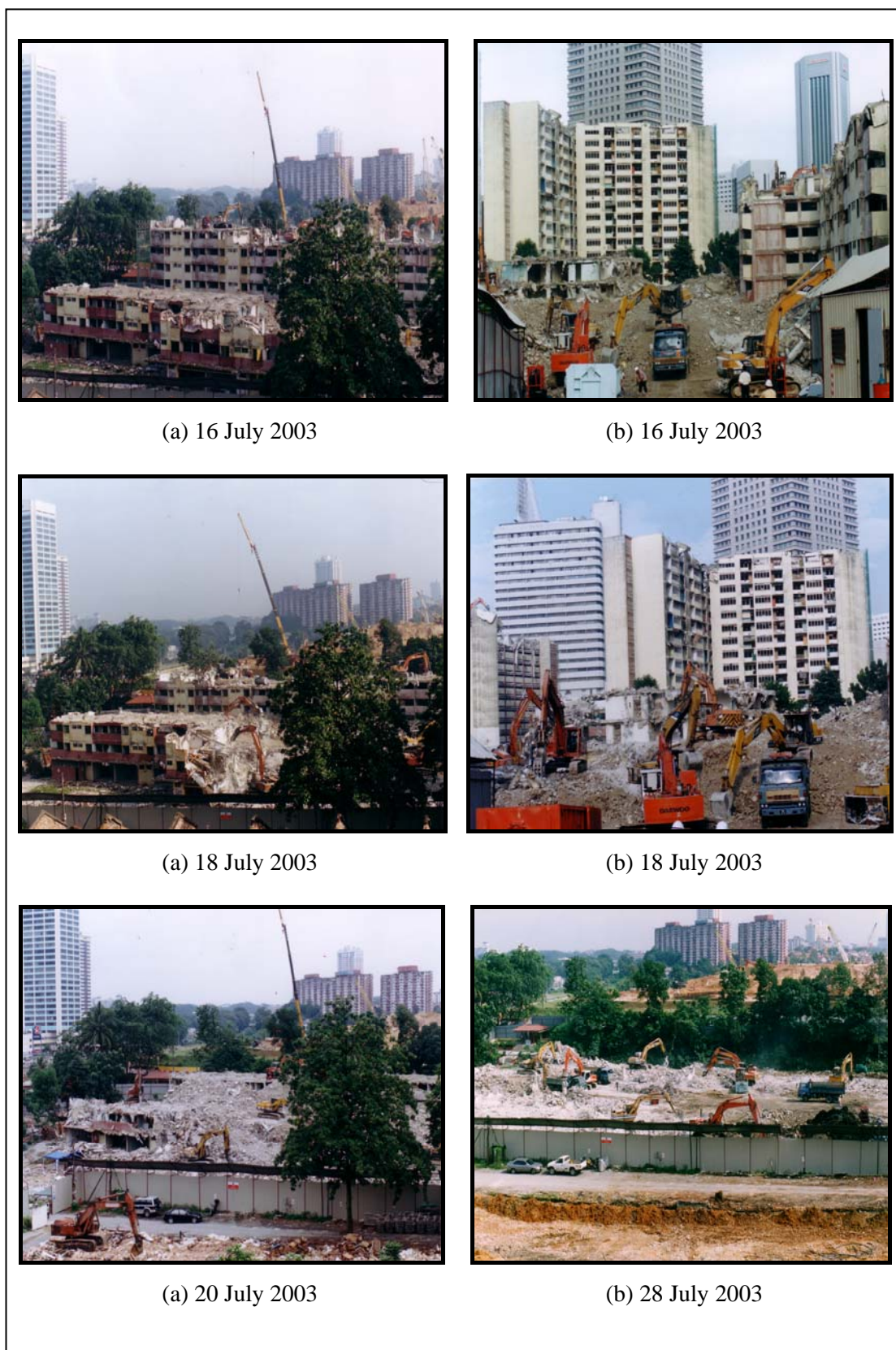
Figure 4.11 (a-f): Demolition operations at Block C.
