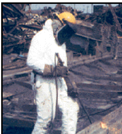
Figure 2.27: Proper protective gear while conducting hot cutting operations (demolitionx.com, 2005).
