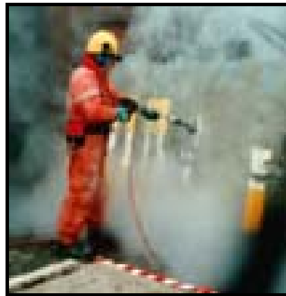
Figure 2.26: Hand operated pressurized water jetting (conjet.com, 2005).
