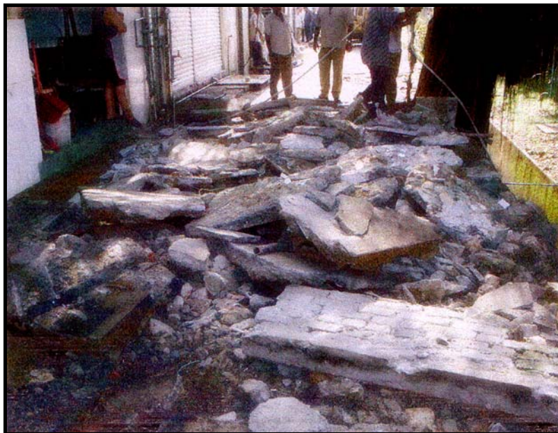
Figure E3 (a-b): Demolition works in progress on an illegal slab extension over the back lane of a shop lot. The works were executed under the authority of Majlis Perbandaran Petaling Jaya.
