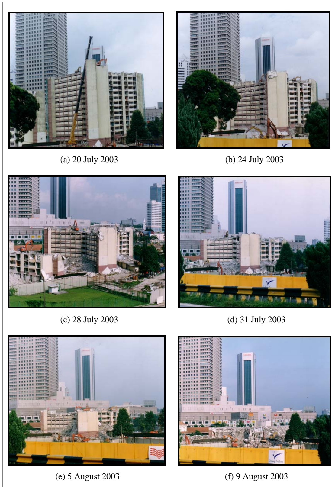
Figure 4.9(a-f): Demolition operations at Block A.
