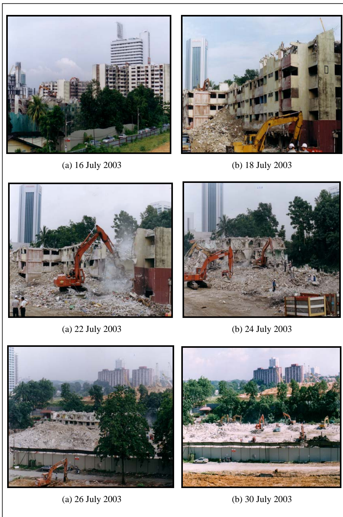
Figure 4.12 (a-f): Demolition operations at Block D.
