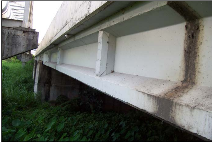
(a) Longitudinal View of the Bridge
