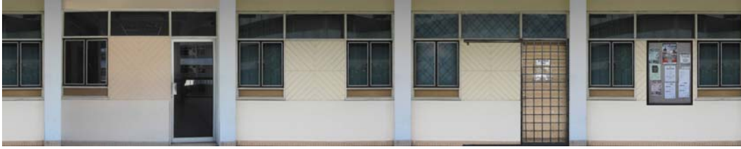
Figure 4.3 Part of the joint rectified photos
