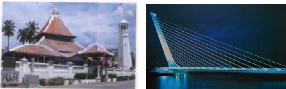
Masjid Kg Hulu-Melaka & Amalino Bridge by Santiago Calatrava
