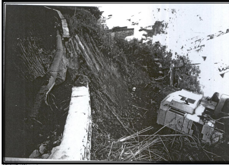
Figure 1.3: Water flowing into the landslide was diverted using PVC pipe
