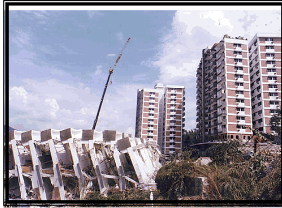
Figure 2.5: The collapse of Block 1 Highland Tower Condominium in 1993. (Source: Berita Harian Online)
