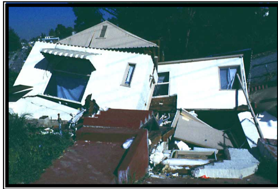
Figure 2.2: House damage after landslide (Source: U. S. Geological Survey, 2001)
