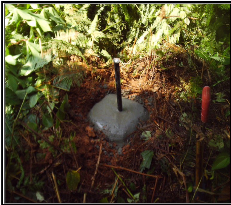
Figure 3.23: Plastering the monument with concrete
