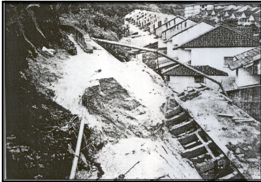
Figure 1.2: Landslide behind the terraced at a double storey houses in 26 th April 2001.
