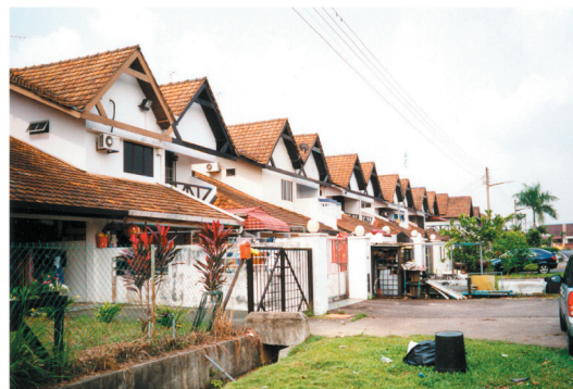
Fig.1. Terraced House Area
