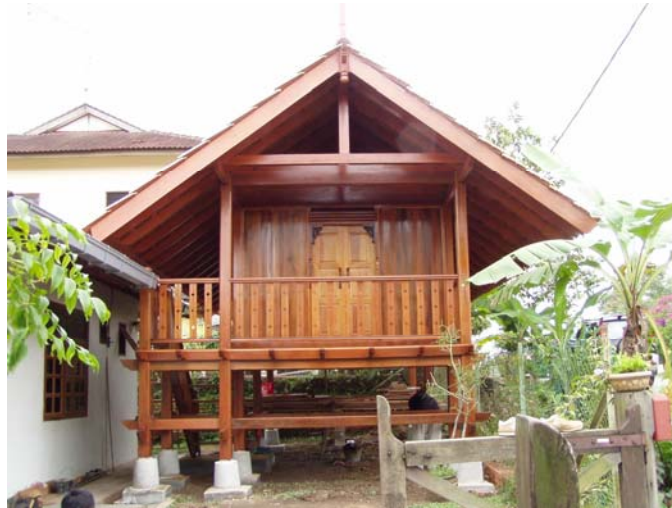
Figure 2: Front view of the timber library.
